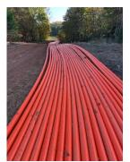
Twenty four individual strands of HDPE conduit were installed at the same time for a new data center.
