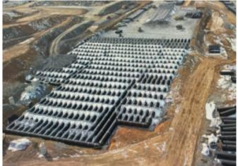
The largest of five retention beds was constructed from 24,500 ft (4.64 miles) of 60-inch diameter corrugated HDPE pipe. Photo shows the bed 50 percent completed.
