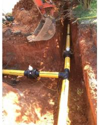
Frontier Natural Gas used more than 50,000 feet of the new pipe in its 100-psi gas distribution system.
